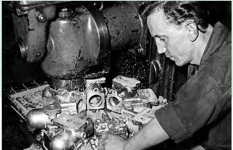
**RESUMPTION OF FILTER PRODUCTION** / In the first few years after 1945, filters were still produced in a large number of individual steps.
