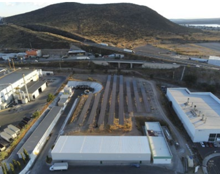
Photovoltaic plant at the site in Querétaro, Mexico
